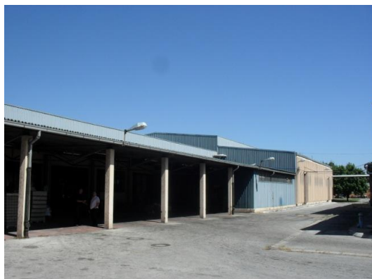
Business complex in Požega
