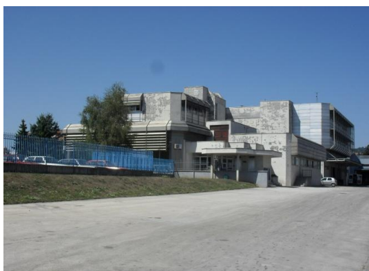
Administarive building in Požega
